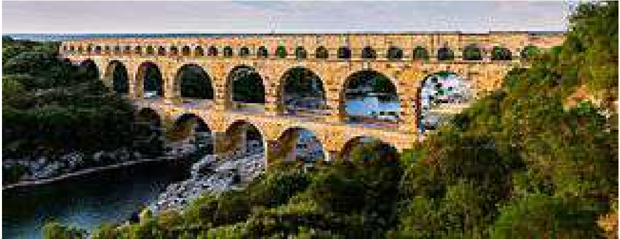
Figure 1.28: A Roman aqueduct: The multiple arches of the Pont du Gard in Roman Gaul (modern-day southern France). The upper tier encloses an aqueduct that carried water to Nimes in Roman times; its lower tier was expanded in the 1740s to carry a wide road across the river.
