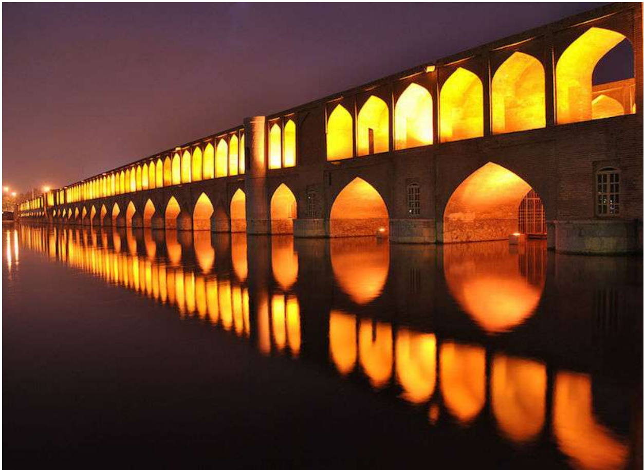
Figure 5.15: Si-o-se Pol (The Bridge of 33 Arches) is a famous bridge in the Iranian city of Isfahan. It is highly ranked as being one of the most famous examples of Safavid bridge design. Commissioned in 1602 by Shah Abbas I, the bridge is build of bricks and stones. It is 295 meters long and 13.75 meters wide. It is said that the bridge originally comprised 40 arches however this number gradually reduced to 33.
