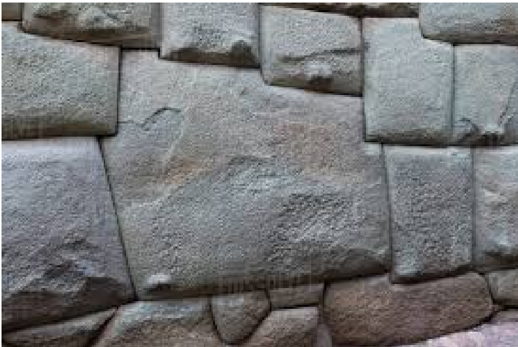
Figure 1.22: Incan stonework. It is impossible to fit a knifeblad between the stones. We do not know how they achieved this degree of accuracy in cutting the blocks.
