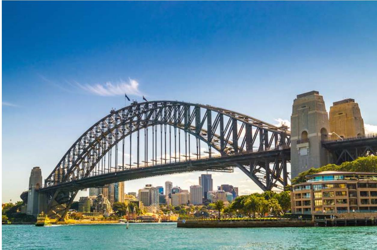
Figure 5.18: Sydney Harbour Bridge is one of Australia's most well known and photographed landmarks. It is the world's largest (but not the longest) steel arch bridge with the top of the bridge standing 134 meters (440 feet) above Sydney Harbour. It took eight years to build and opened in March 1932. Because the steel expands or contracts depending on whether it is hot or cold the bridge is not completely stationary and can rise or fall up to 18 cm (7.1 inch).
