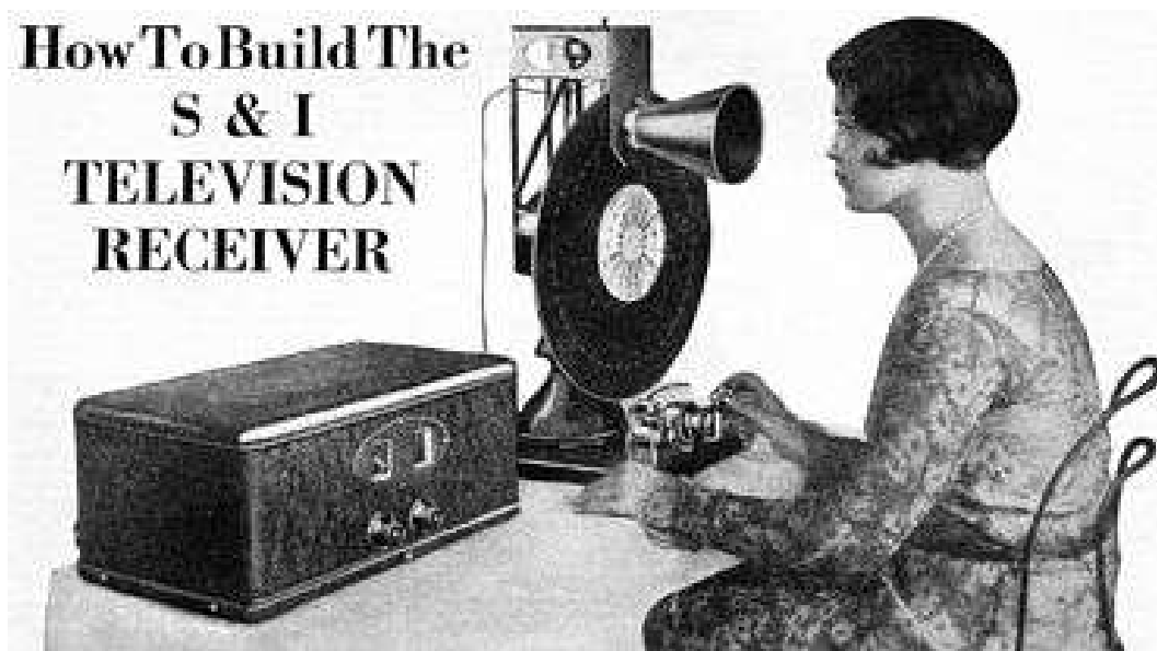
Figure 9.4: Watching a homemade mechanical-scan television receiver in 1928.
