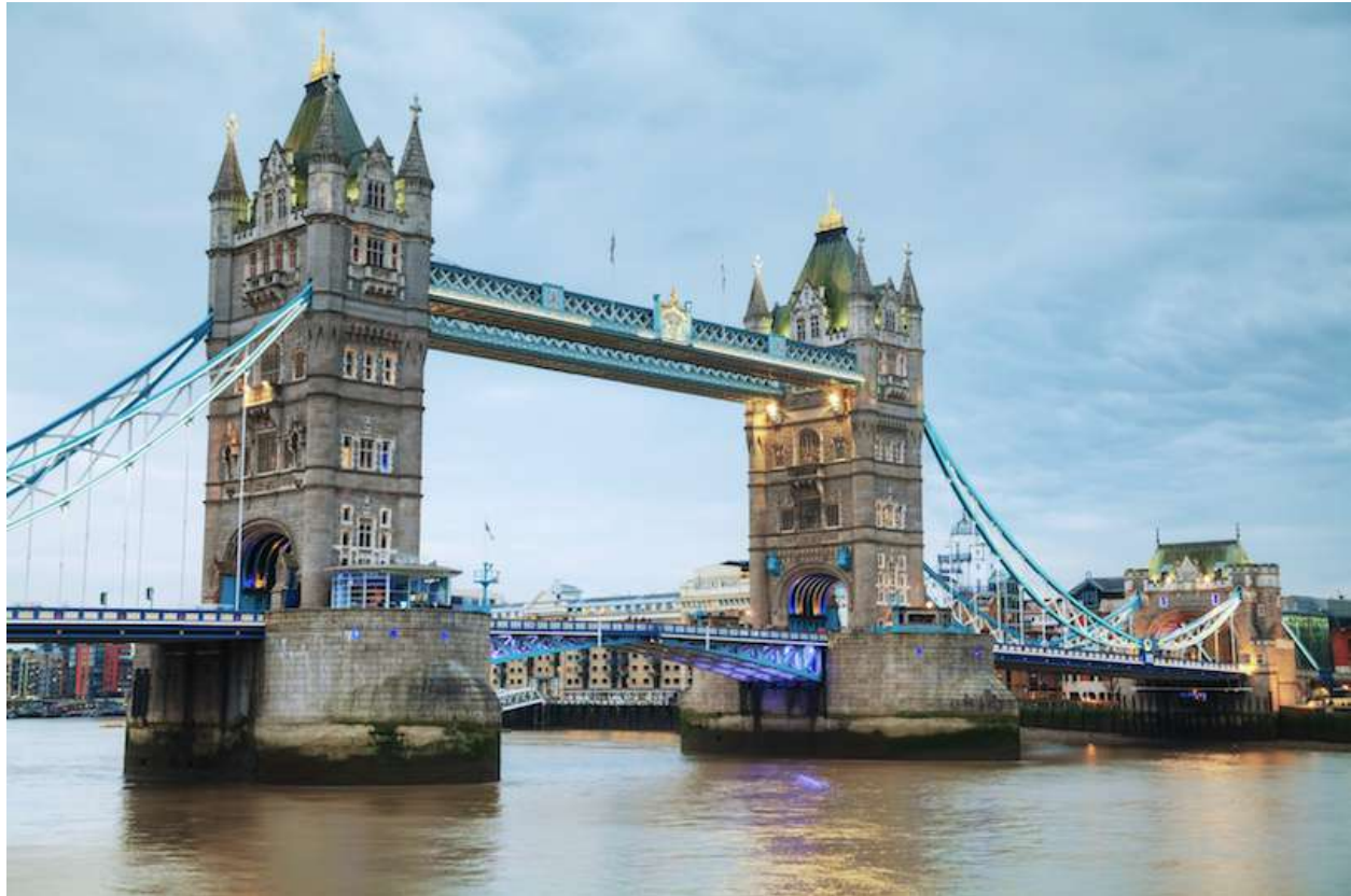
Figure 5.16: Tower Bridge is a combined bascule and suspension bridge in London, over the River Thames. It is close to the Tower of London, which gives it its name and has become an iconic symbol of London. Construction started in 1886 and took eight years to build. The bridge consists of two towers which are tied together at the upper level by means of two horizontal walkways which are designed to withstand the forces of the suspended sections of the bridge.
