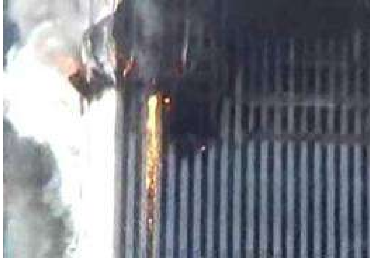
Figure 3.9: Molten steel pouring from one of the twin towers before its collapse.
