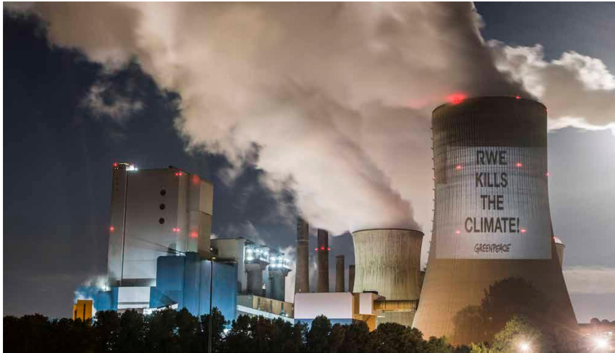
Figure 3.9: A coal-fired power plant.
