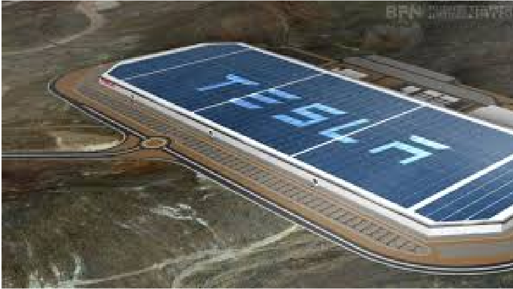
Figure 2.25: Tesla's Gigafactory 1 in Nevada produces improved lithium ion batteries. Energy for the factory is supplied by solar panels on the roof.
