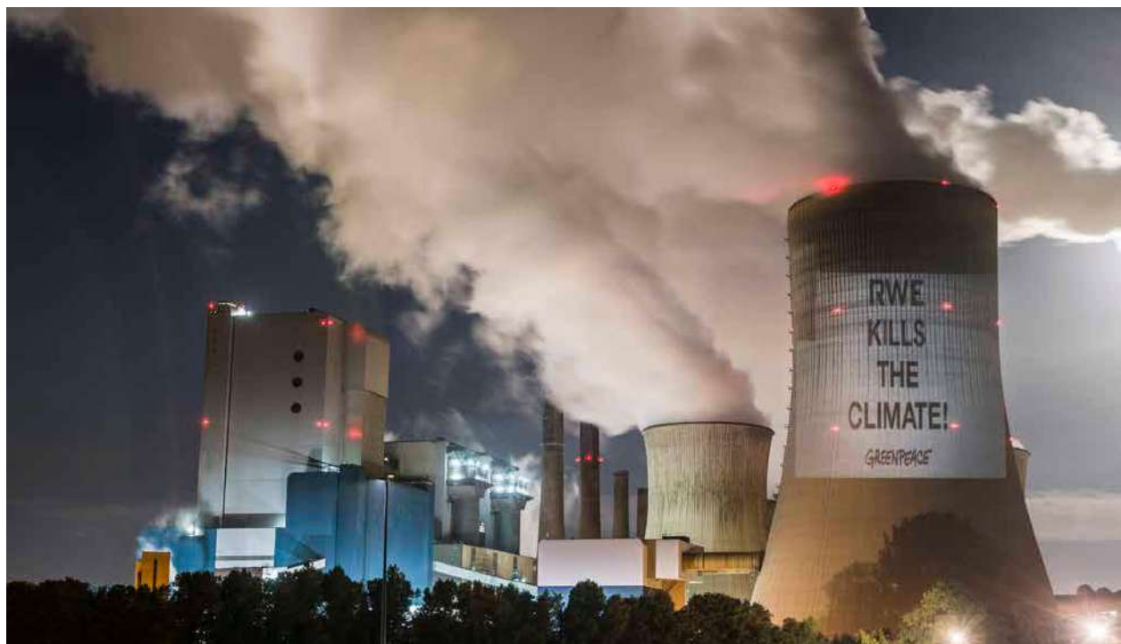
Figure 2.48: A coal-fired power plant.
