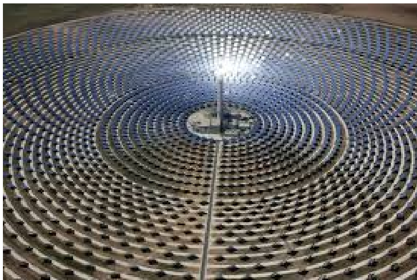
Figure 2.3: A solar thermal power plant. Arrays of heliostatic reflectors concentrate the sun's rays onto molten salt in the tower. The plant produces electricity at night because the salt remains hot..
