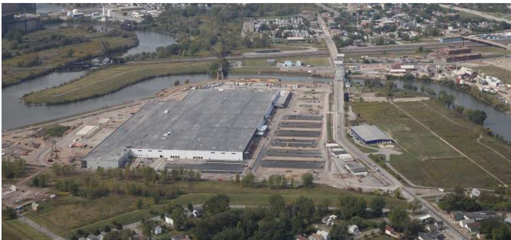
Figure 2.26: Gigafactory 2. SolarCity's factory in Buffalo New York produces high-efficiency solar modules. Elon Musk estimates that only 100 gigafactories would be enough to achieve a worldwide transition to 100% renewable energy.
